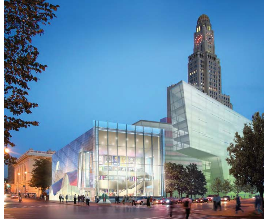
Figure 1.9 – A rendered CAD image for the Theater for a New Audience in Brooklyn, New York. All the elements in the scene are modeled with geometry and rendered using materials, textures, lighting effects (including shadows, reflectance, transparency, etc.), and atmospheric effects (sky and haze) to achieve realism. (Image courtesy of H 3 Hardy Collaboration Architecture LLC, New York, NY)
