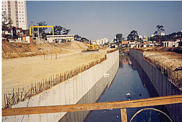
Figure 4.1: Avenue Roberto Marinho Works, with Stream Infrastructure
