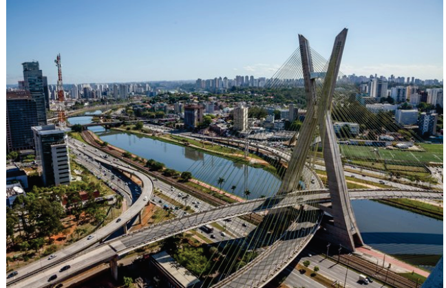
Figure 4.2: Octavio Frias de Oliveira Bridge (Cable-Stayed Bridge)
