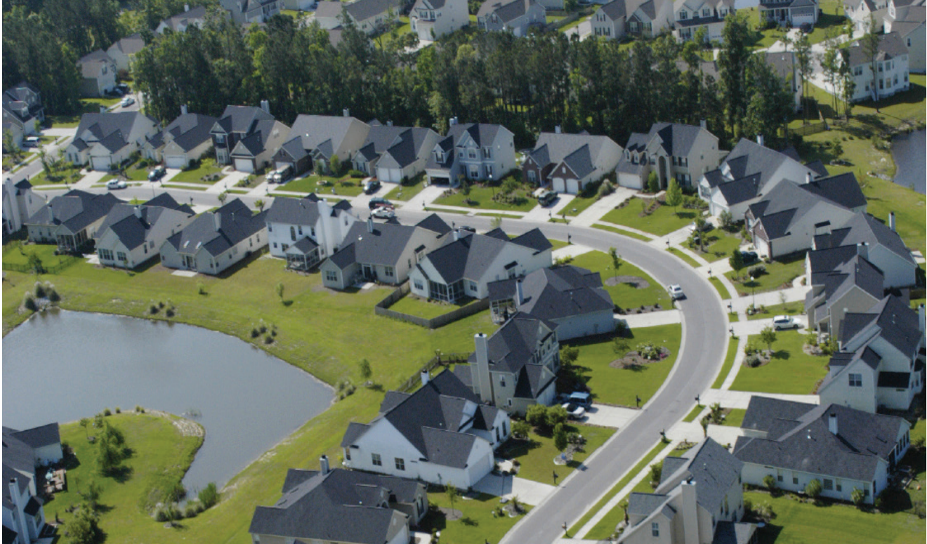
Aerial view of homes in a large residential community. Photo: iStock (2003).
