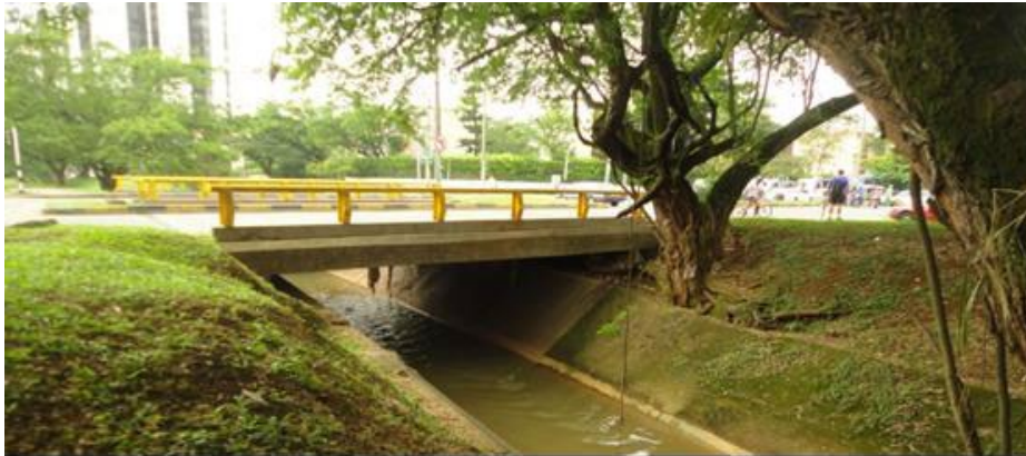
Image 6: Cañaveralejo Canal (Case Study Area's Canal Part, Zone 5 from Image 3 Above).
