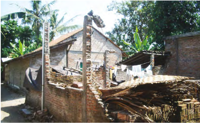
In Yogyakarta, new homes were constructed adjacent to those that were damaged by the 2006 earthquake. Source: R. Olshansky (2008).
