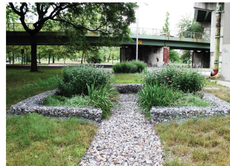
A Highway Overpass Landscape Detention (HOLD) System is a modular bioswale that can be deployed under elevated infrastructure to filter and retain excess stormwater. Photograph courtesy of DLANDstudio Architecture + Landscape Architecture, PLLC.
