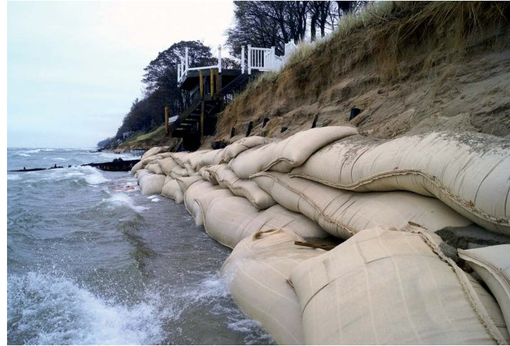
To protect against storms and flooding, Grand Haven provides sandbags and sand to property owners. Credit: Courtesy of Grand Haven Charter Township.
