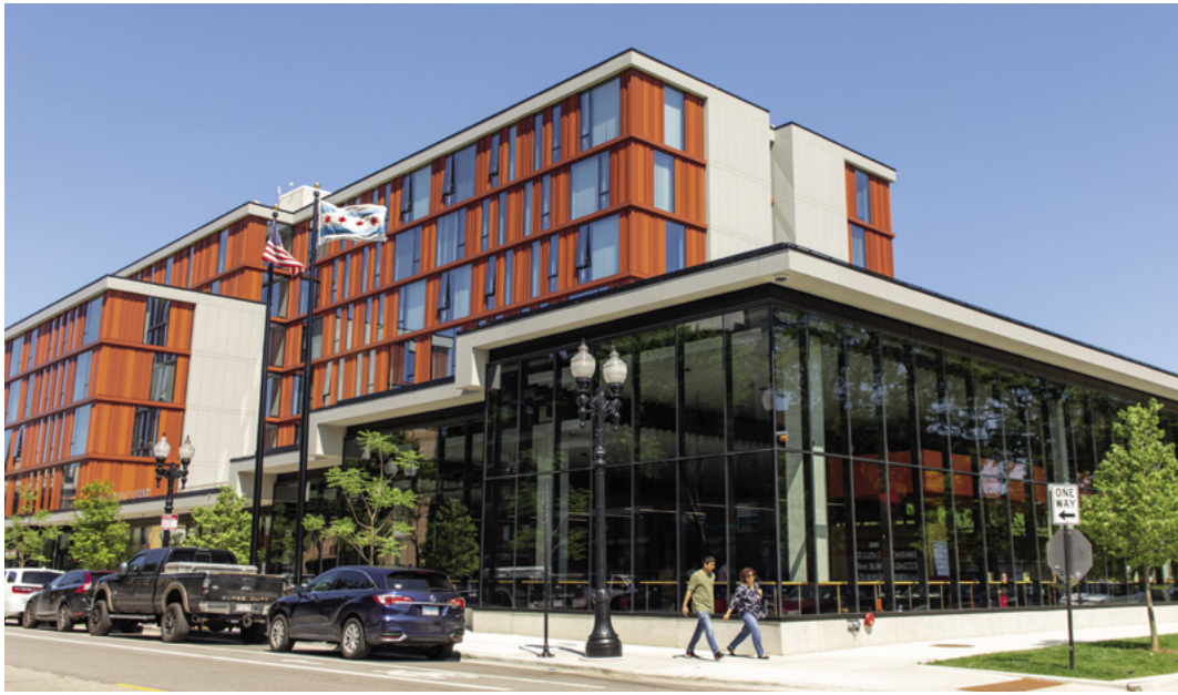
A mix of sources covered the cost to build the award-winning Little Italy Branch Library and Taylor Street Apartments in Chicago, including federal funds, tax credits, and TIF revenue. Credit: Courtesy of Chicago Housing Authority.
