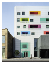
Independence Branch Library and Apartments in Chicago, a mixed-use development that combines a public library with affordable housing. Credit: James Florio, courtesy of John Ronan Architects.
