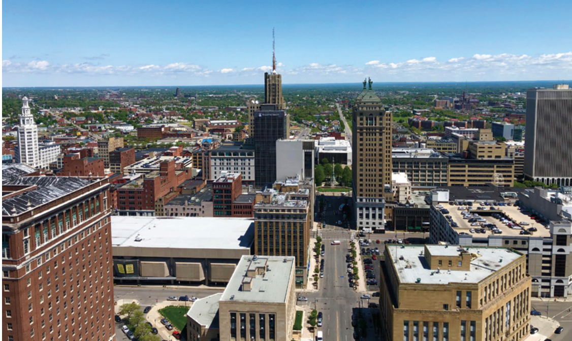
The city of Buffalo, New York, is investing in green infrastructure projects including porous pavement, bioswales, and green roofs. Credit: Andy Rosenblum via iStock/Getty Images Plus.
