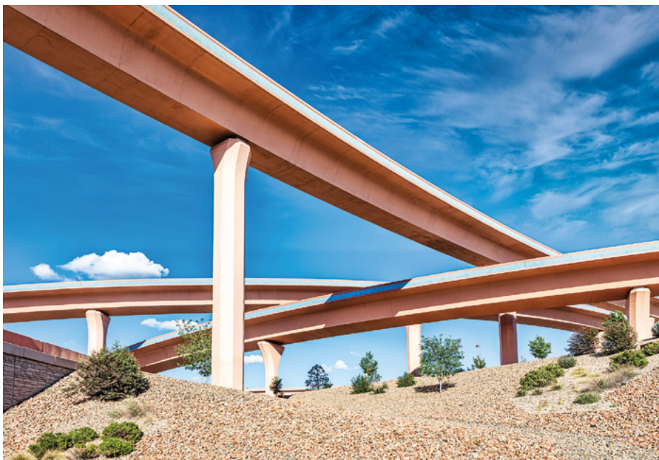
The construction and management of major infrastructure projects like highways, such as this interchange in Albuquerque, New Mexico, requires cooperation between federal and state governments. Credit: Mlenny via iStock/Getty Images Plus.
