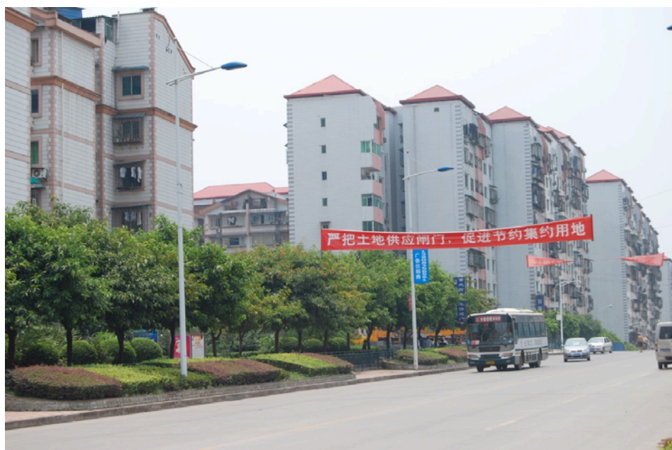
Figure 5. New Housing Estates for Relocated Rural Residents—Hemulu Neighborhood
